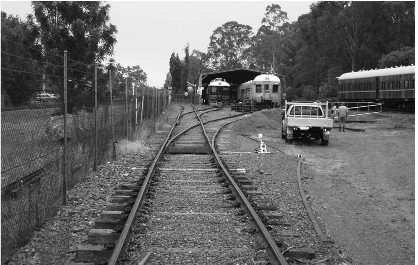
The rebuilt track work taken from the same location in February 2009.
