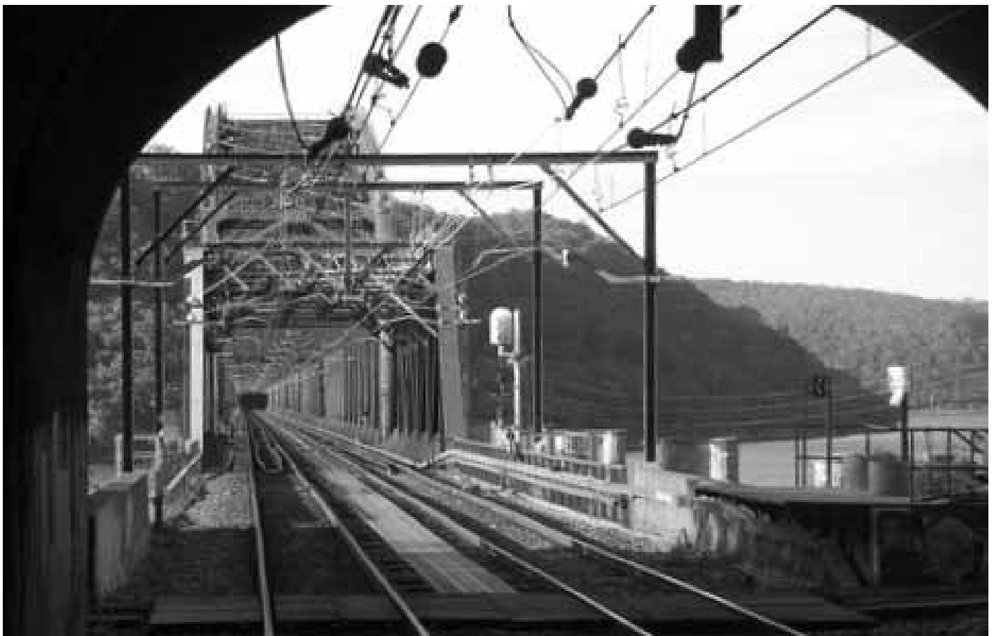
Exiting Long Island tunnel approaching Hawkesbury River bridge.
