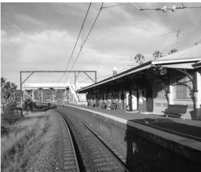
Down platform Hawkesbury River.
