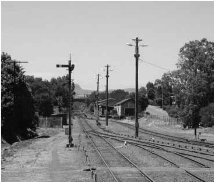
Up starting signal and derelict goods sheds Bomaderry.
