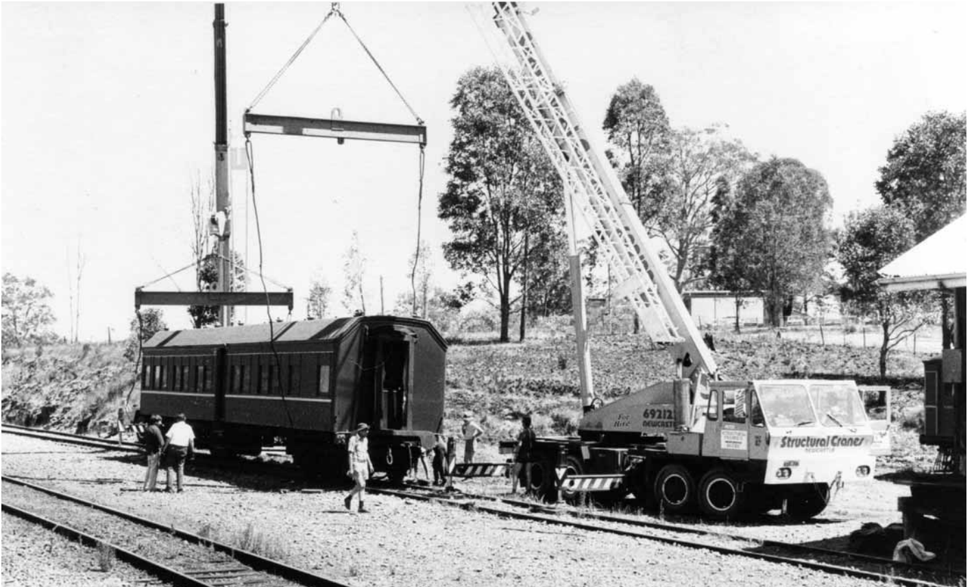
The crane lift on 10th October, 1984 was planned to utilise the two hired mobile cranes as economically as possible so that the whole operation could be accomplished in one day. The second lift was to place BRI395 on its own bogies on two short sections of track parallel to the goods line and inside the proposed boundary fence line. Photo: Geoff Murray
