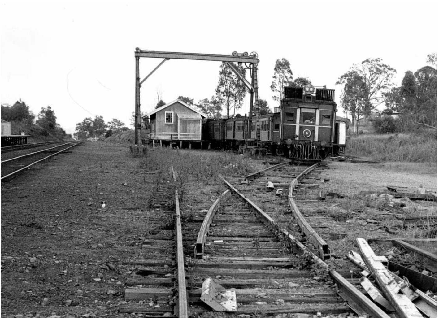
After an epic journey from Sydney, the six CPH's are safely stowed on No.1 road at Paterson. The temporary turnout can be seen in position in the foreground.
