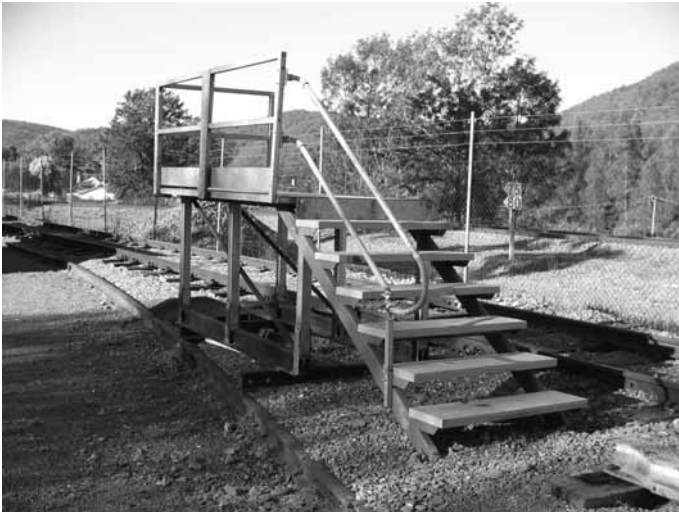
Depot platform under construction.
