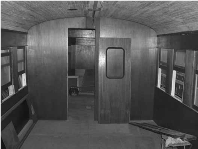
New varnished internal linings completed and ceiling ready to re-paint.
