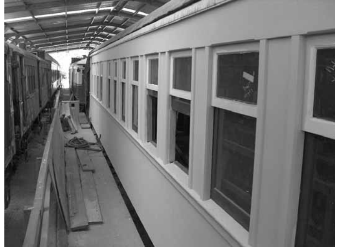
Completed side fitted with new windows and crownlights.
