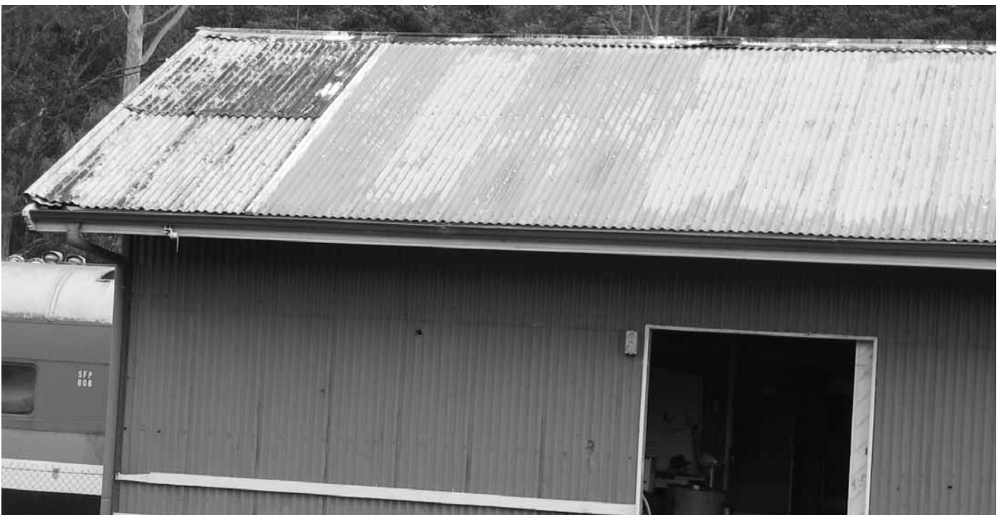
Re-roofing the goods shed in progress.
