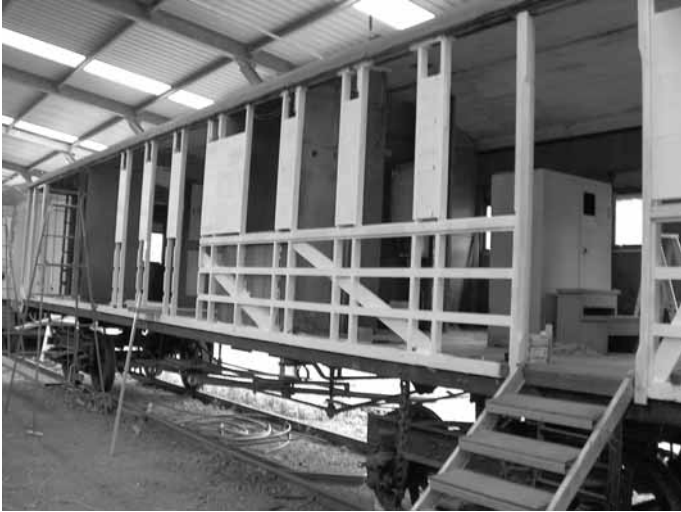
New side framework under construction.
