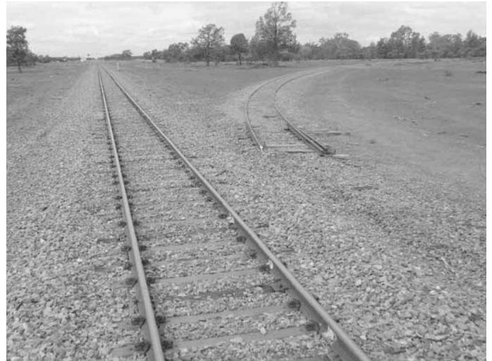
The disconnected western leg of the triangular junction to the Parkes – Broken Hill line at Roto. This was once the connection to the cross-country line to Griffith and Narrandera. Photo: Peter Larkins
