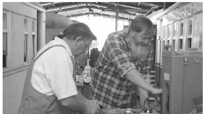
621/721: With the October long weekend tour to Gulgong fast approaching, carriage builder Alwyn Williams (left) assisted by Warren Mills (right) and Stephen Davies have been preparing catering facilities similar to those in the CPH's.
