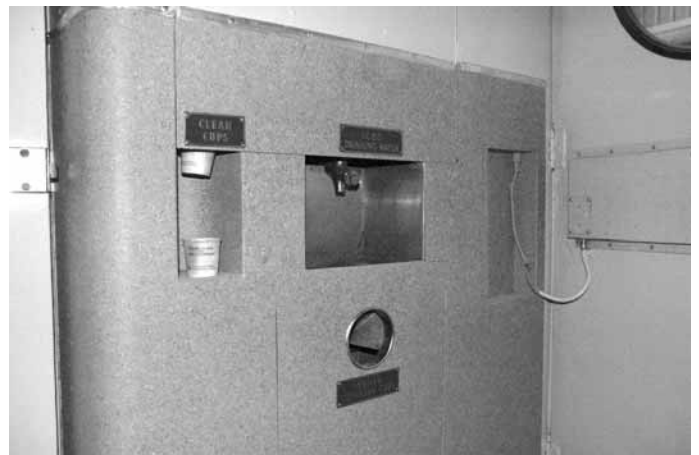
Hidden behind a steel panel for years the original Iced Water unit has now been restored and is ready for another service career.
