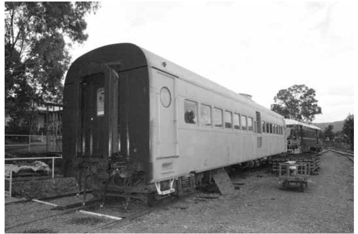
External priming of power car 629 has been completed and some test painting conducted on the vestibule end to check final paint colours.
