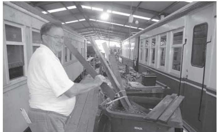
Alwyn Williams soaking roof laths for CTC 51.
