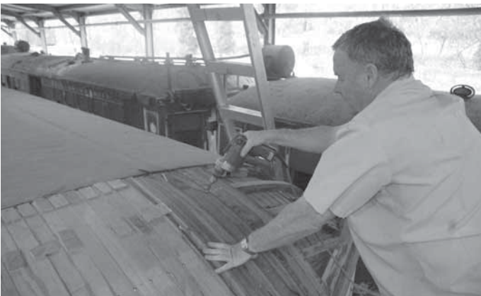
Stephen Davies attaching new roof laths.
