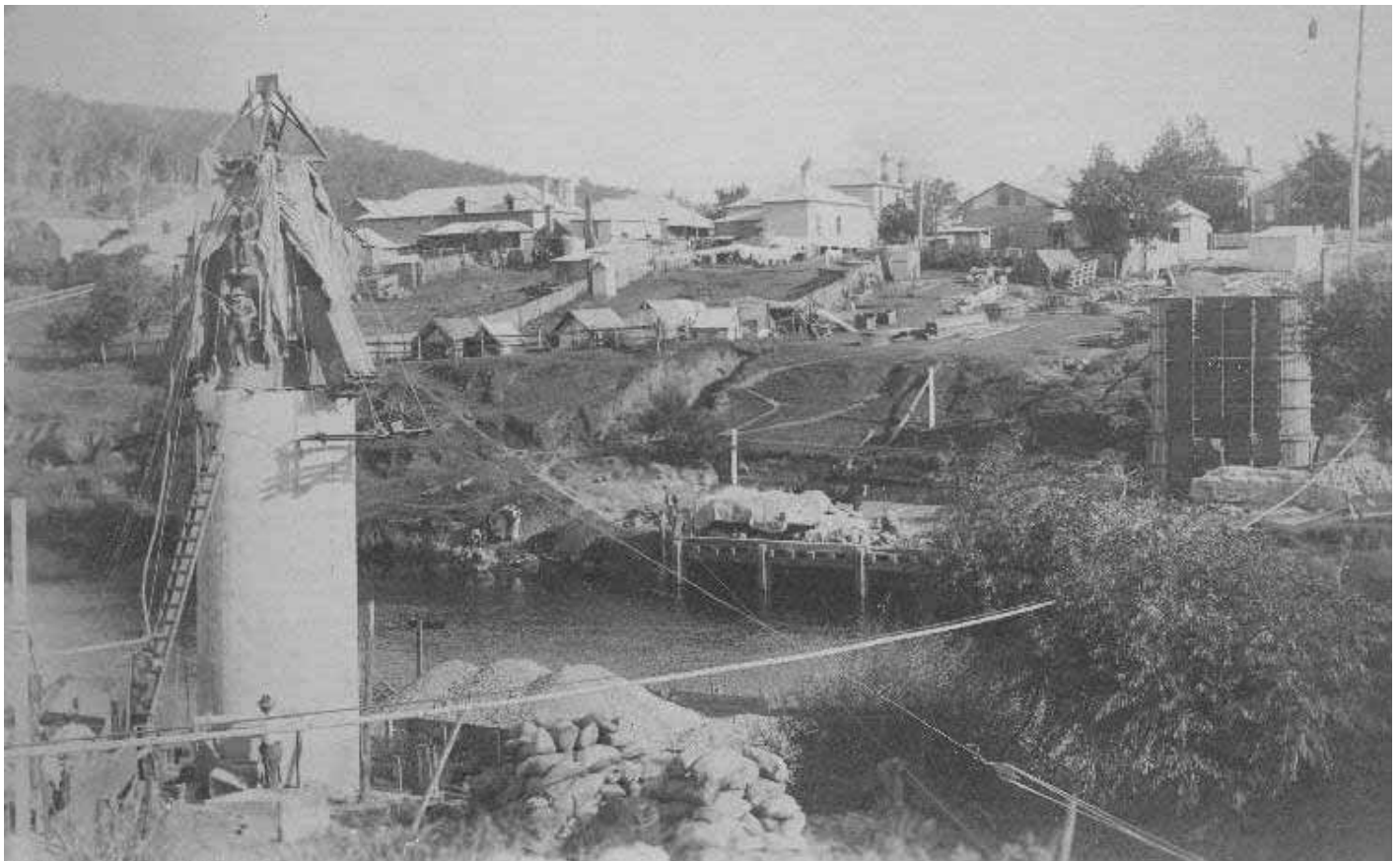
Paterson railway bridge under construction, circa 1909.
