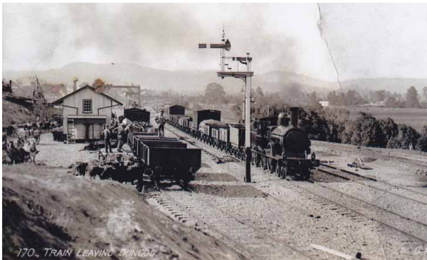
This early view of Dungog (circa 1912) shows an Up mixed train hauled by a D255 (later 15 class) locomotive headed for West Maitland while in the goods yard much activity is underway transshipping goods. Unusually for the times, the loading hands have not paused to watch the camera and with several horse and bullock drawn vehicles queued they are obviously focused on their hard manual tasks at hand. Of note is the still immaculate presentation of the yard and infrastructure including the magnificent McKenzie and Holland bracketed signal post complete with somersault arm for loop line movements.
