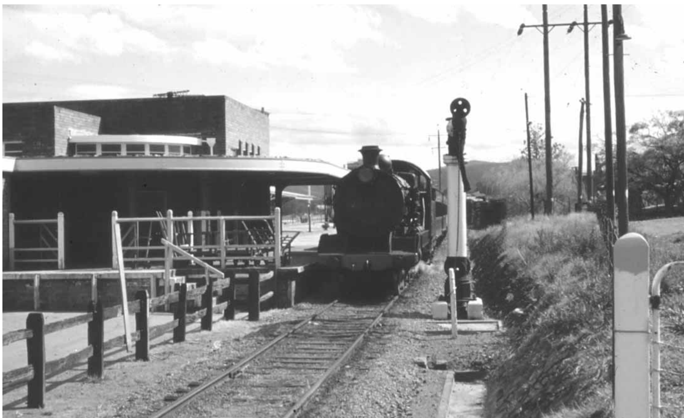
This 1960's shot of Dungog's back platform road features the once regular sight of a 35 class steam locomotive hauled passenger service, the obligatory water column to replenish the engines tender and the original loading dock arrangement for station parcel delivery and collection by lorry. Photo: R. G. Preston
