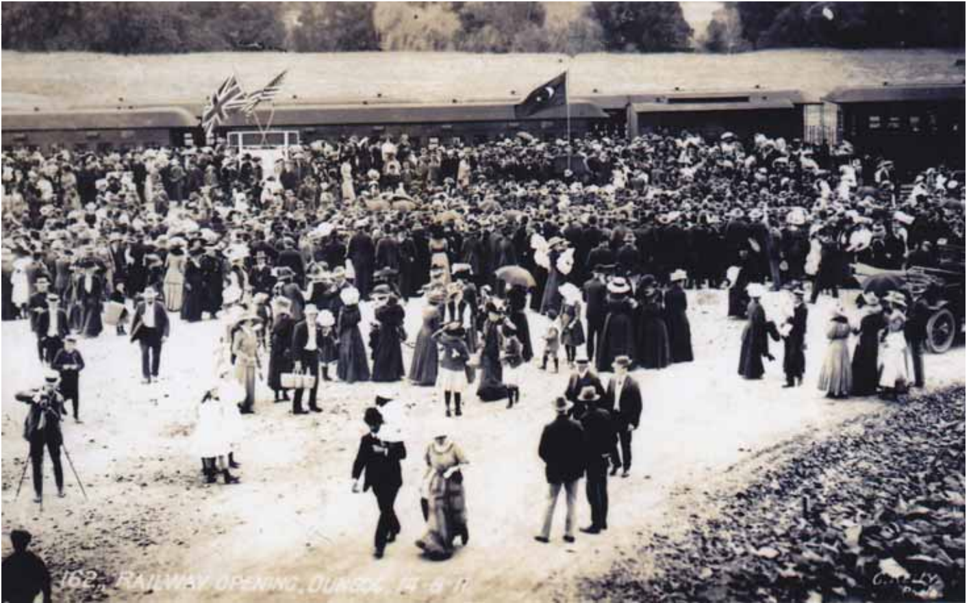
The opening day of the railway to Dungog was a cause for much celebration with a good representation of Government officials, local dignitaries and towns folk attending the festivities. Dressed in their Sunday best the large crowd is seen here assembled in the Dungog station entrance and platform area watching the opening ceremonies, standing behind on the Main line and loop are the carriages which formed the two trains run from West Maitland for the occasion. Photo: Dungog Historical Society
