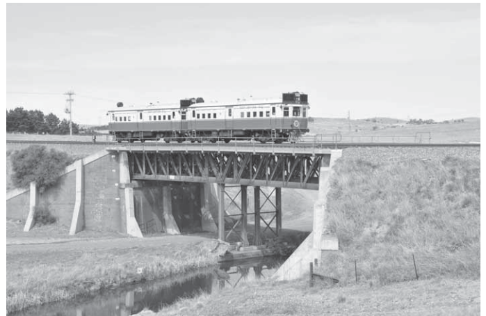
Underway again after a perway delay the CPH's cross the truss bridge at Joppa Junction and commence the climb up to Cooks cutting. Photo: S. Preston
