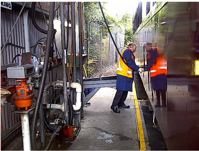
Fred the Fitter attaches the water hose in preparation to decant 721. Photo: S. George
