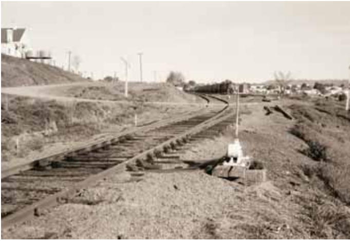
Unlike the entrance to most country yards, Barraba had no interlocking equipment and relied on point clips to provide the mandatory locking for the passage of passenger trains. High on the hill the Station Master's cottage overlooks the yard with its unprotected entrance, level crossing and simple but sufficient track layout.
