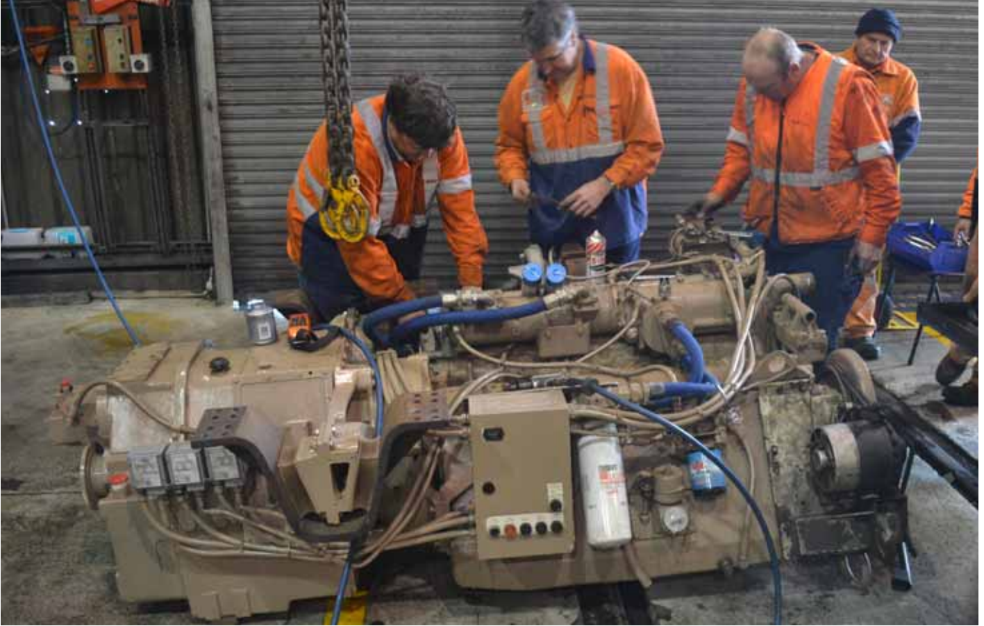
The team from Broadmeadow ESC prepare the new engine and transmission for installation.
