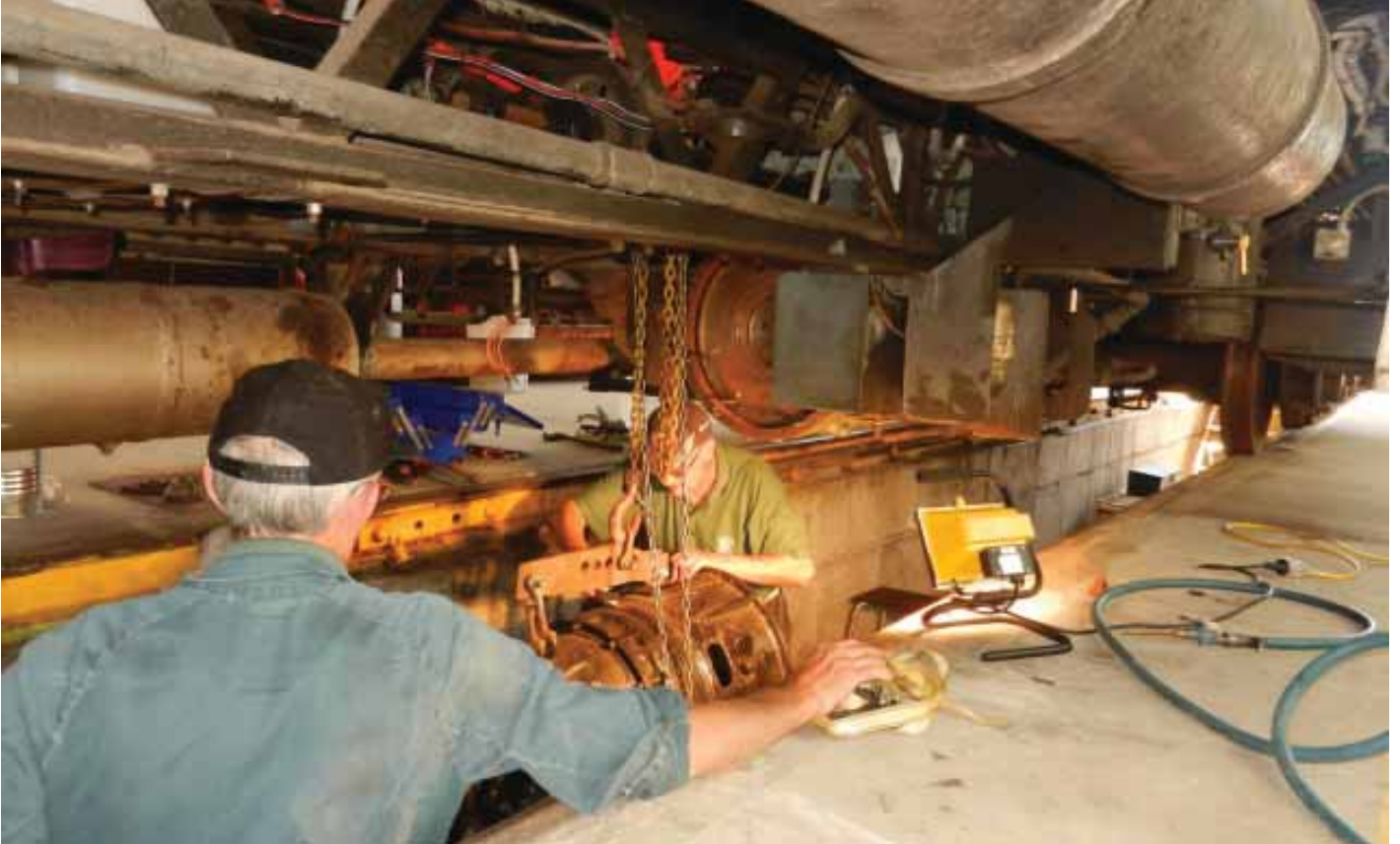
The reconditioned torque convertor installed in CPH 3 in the lead up to its return to traffic was found to be faulty in service. Here Wal Williams stands by to assist Stafford Payne with the installation of a replacement. Photo: Stephen Davies
