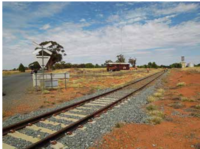
The end of the line at Oaklands has been reached with 402 seen standing clear of the terminus earth mound on the abandoned NSW line from The Rock. The line in the foreground is the former dual gauge siding to the stockyards and Commonwealth siding which although having been provided with concrete sleepers to cross the road finishes shortly after in a ballast mound, the section of track beyond remaining gauged to 5'3".
