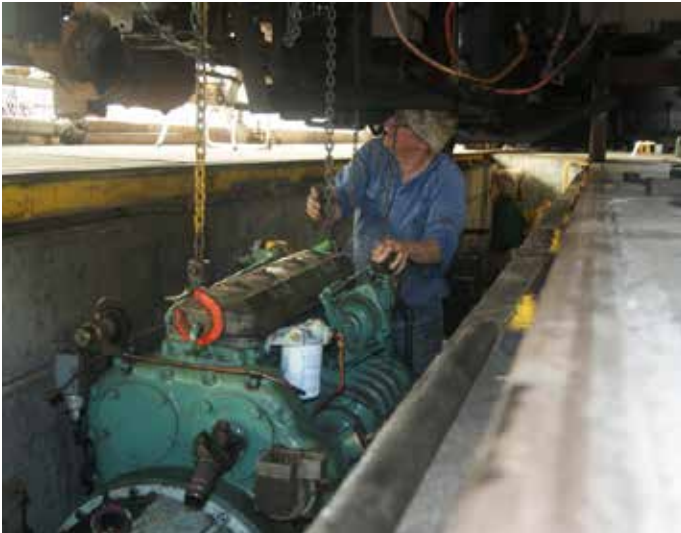
With lifting chains attached to the motor and transmission, Bryan Hicks prepares to watch and guide the lifting process from the service pit below 402. Photo: Steve Davies
