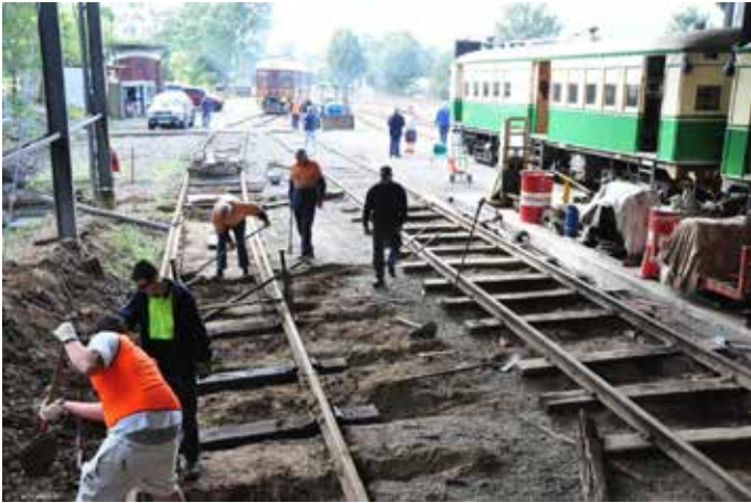
Wednesday work days at Paterson can be busy affairs with all manner of tasks to attend to. On 5 June, not only were preparations underway for the weekend's operations to Nyngan and Oaklands, but replacement of sleepers on No.3 road were undertaken as well as general yard maintenance. Photo: S. G. Preston
