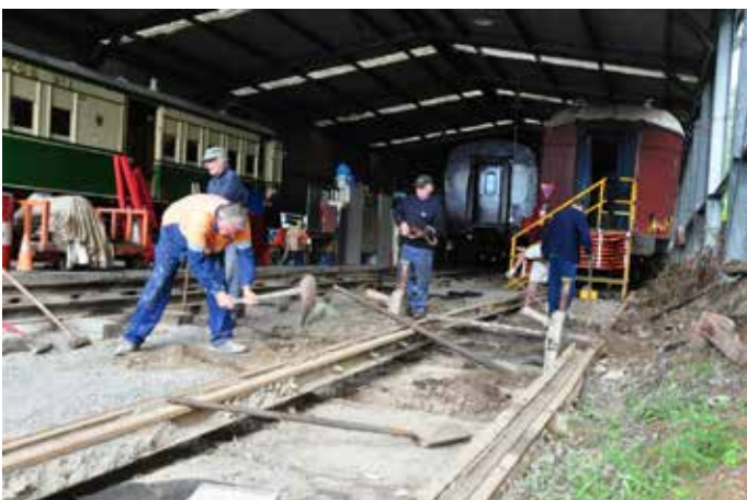
The pelican is in full flight as sufficient spoil is removed from the road bed to allow the positioning of another replacement sleeper. Photo: S. G. Preston
