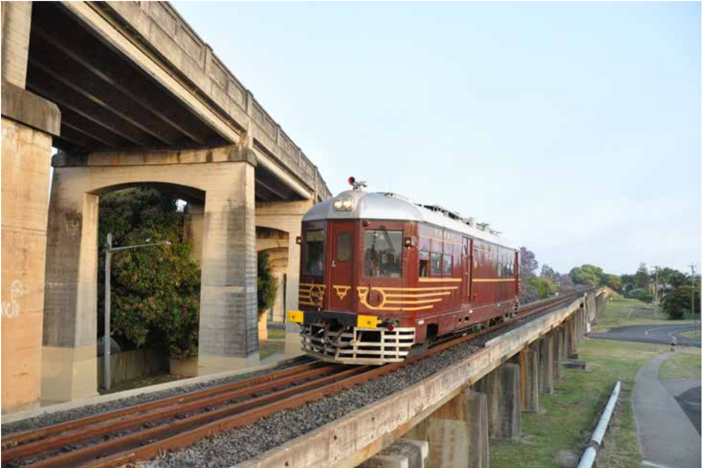
402 rolls along the concrete viaduct approach to Grafton's Clarence River Bridge. The ramp structure in the background elevates the road to pass over the railway on the bridge span shared by both road and rail. Photo: S. George
