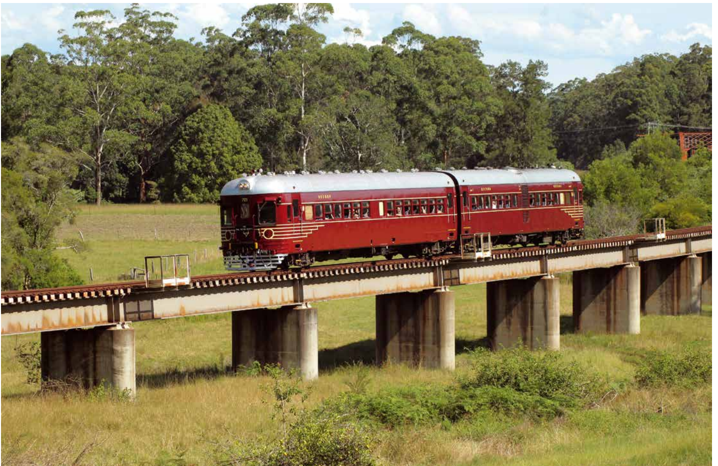
721/621 rolls across the bridge on the approach to Telegraph Point. (Photo: Scott Schache)
