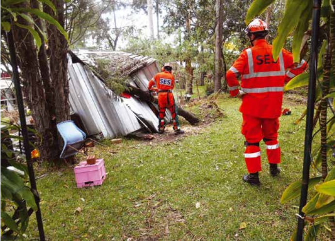
The Society was fortunate that only minimal damage to depot infrastructure occurred during the storms. Ron Pirie's photo above shows SES volunteers cutting a fallen tree which unfortunately landed on and crushed the mower shed.
