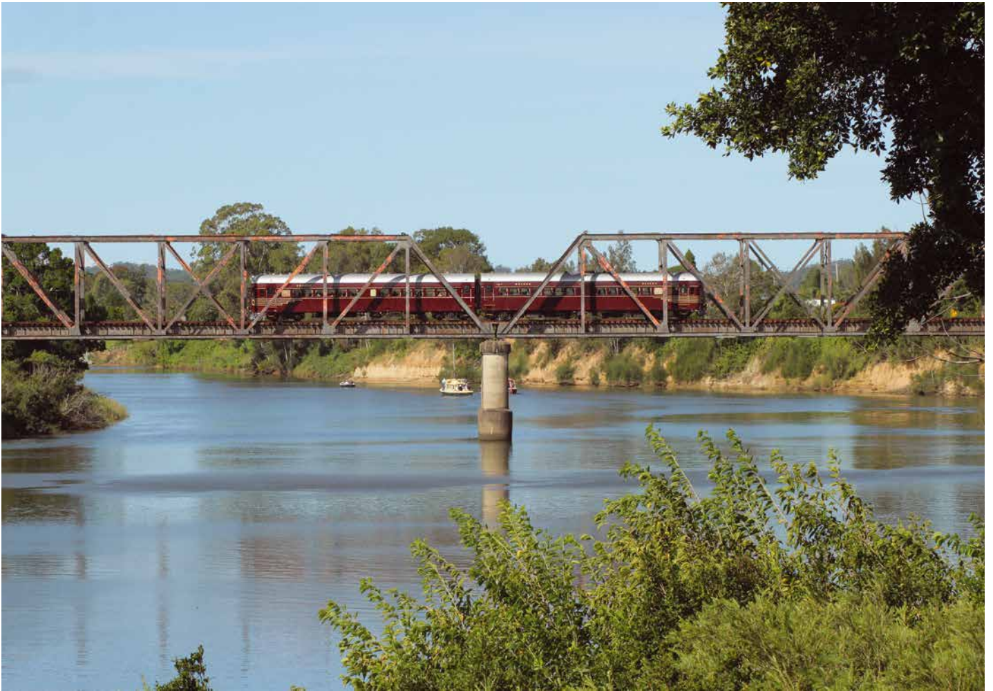
721/621 crosses the Hastings River bridge at Wauchope. (Photo: Scott Schache)
