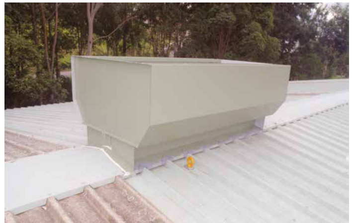
The completed roof ventilator. (Photo: Bruce Kingsford)
