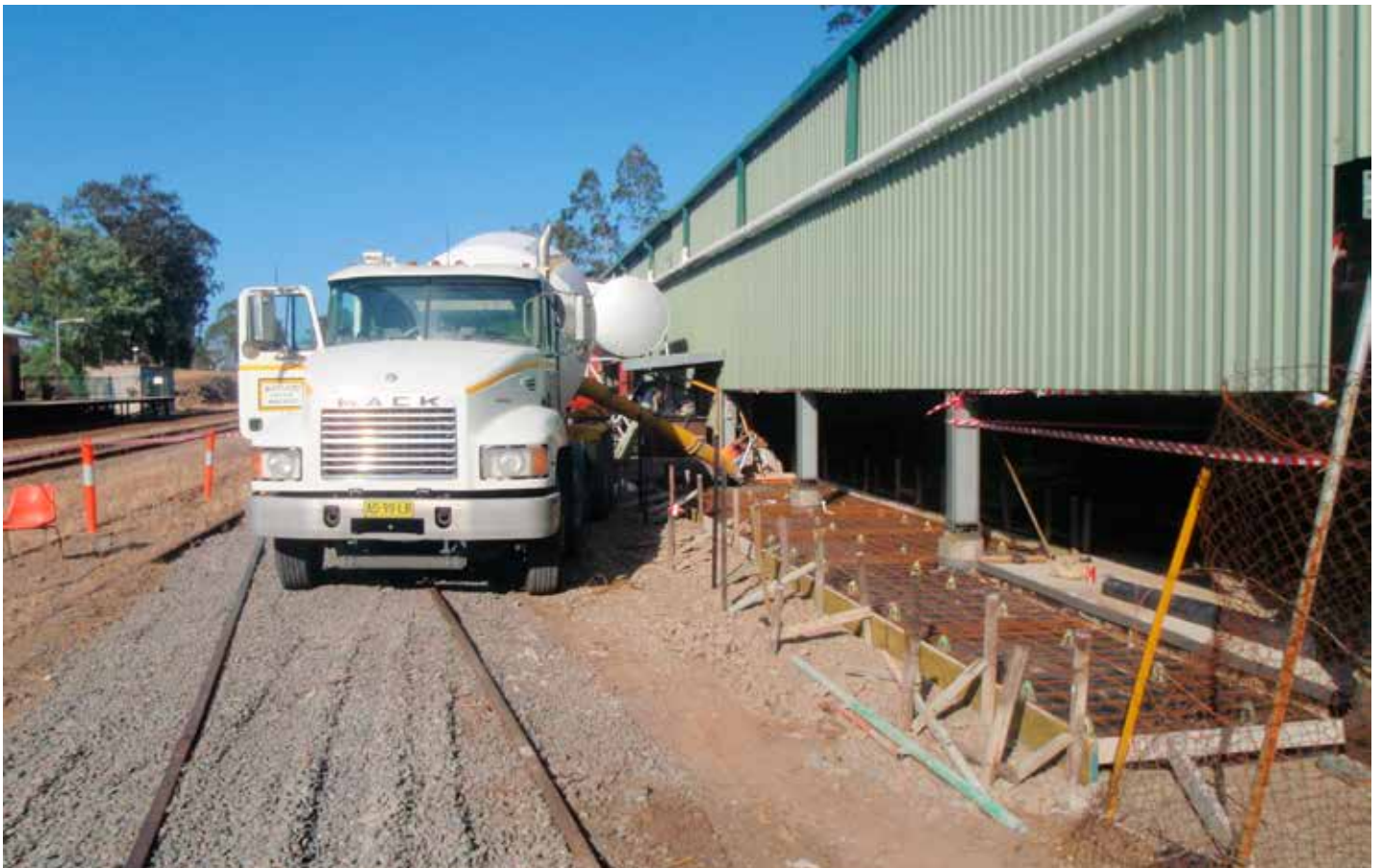
(Above) The frame work required to create this maintenance annex are obvious in this photo looking toward Paterson station. (Below) The formed up annex slab receives the first load of concrete. (Photos: Bruce Kingsford)
