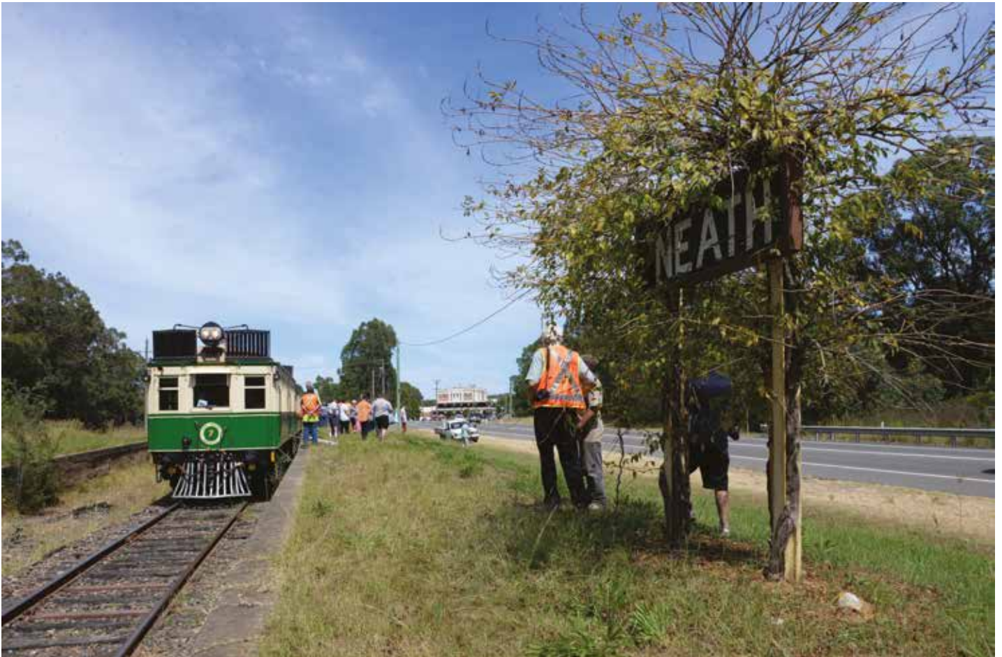
While Neath is no longer an SMR safeworking location many familiar landmarks remain at the station precinct including the Up and Down platforms, station name boards and Signal Box building. Unlike the station, the famous Neath Hotel continues to trade and serve its customers. (Photo: S.G. Preston)
