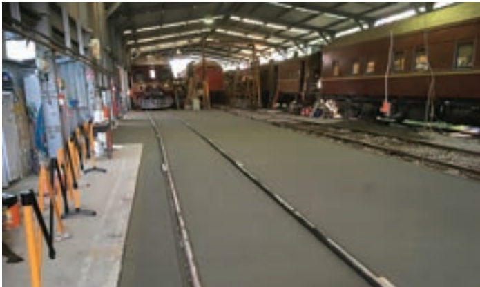
The freshly laid concrete.(Photo Rod Short).
