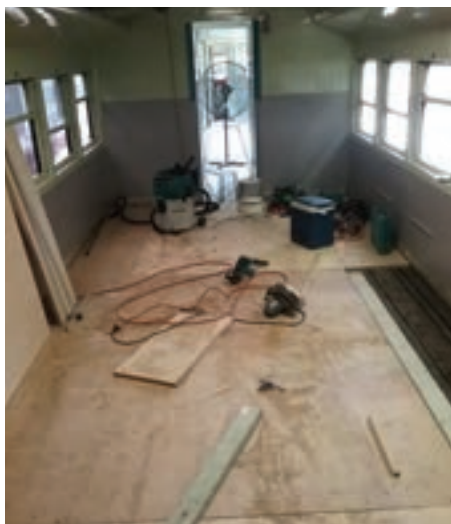
New ply flooring being installed (photo TRMS)
