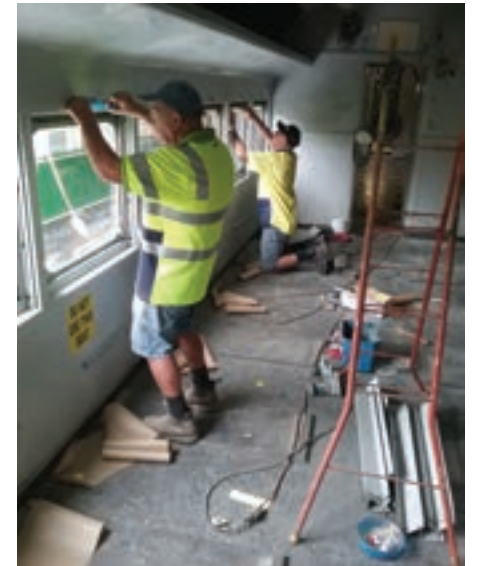
Greg & Bruce masking in preparation for painting (Photo TRMS)
