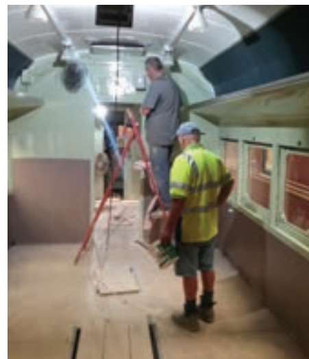
Peter & Greg apply finishing touches (photo TRMS)
