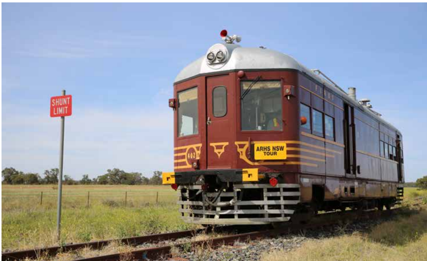
402 is seen here at the current limit of travel on the Warren South branch. Ahead a bridge lies burnt out. (Photo: Robert Spencer)
