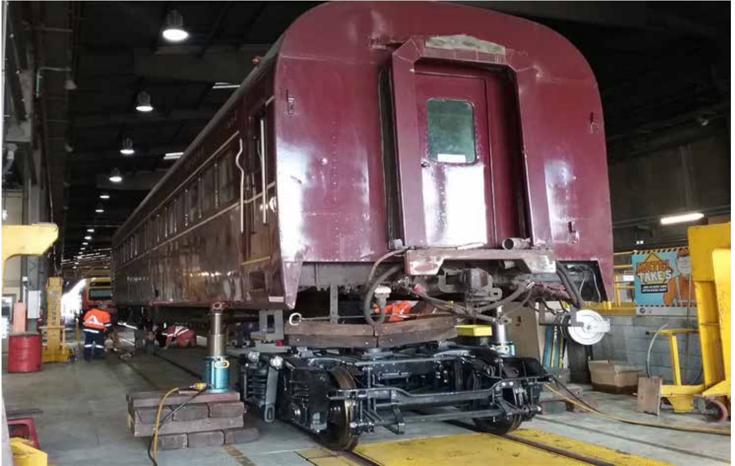
A new rear bogie has been positioned under 721, awaiting connection when the car is lowered. (Photo: Mick Walsh)
