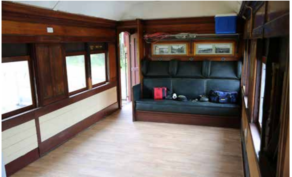
New flooring has been laid in the BR carriage.
