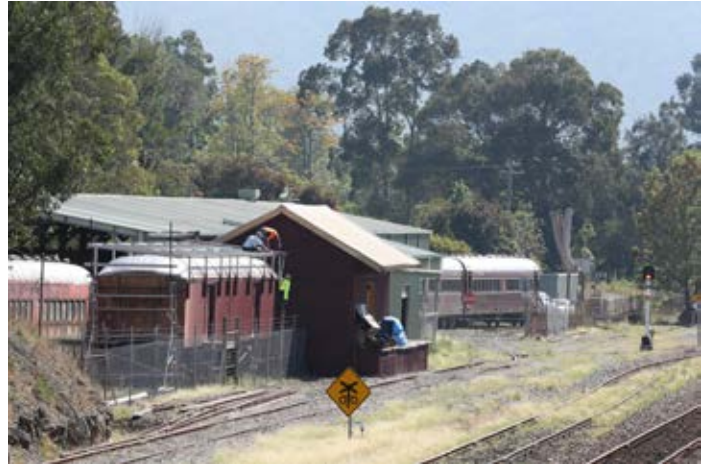
Work commences on fitting roofing sheets to the frame
