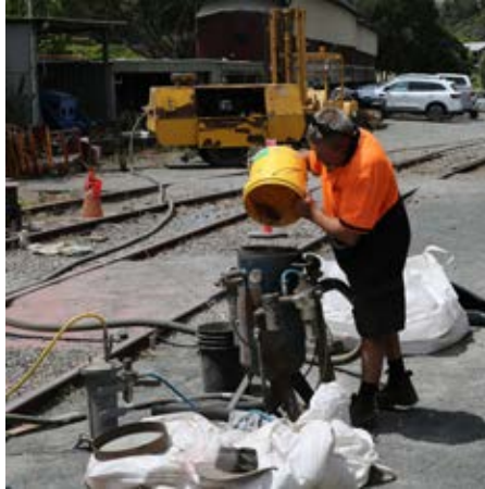
Graeme Holloway maintains feed to the sandblaster
