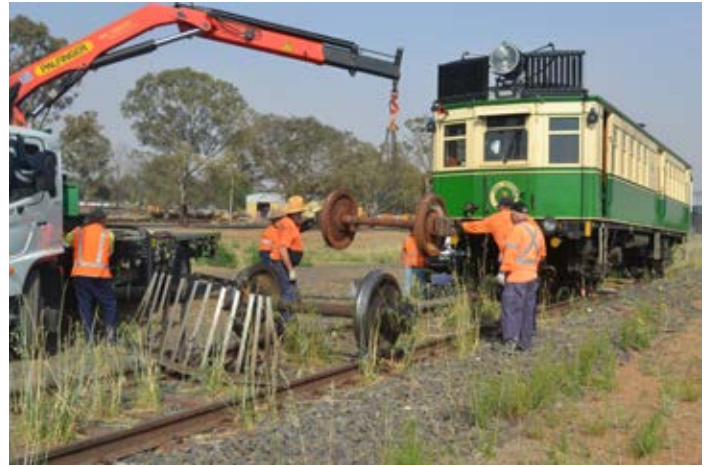
(2) New axle being lowered
