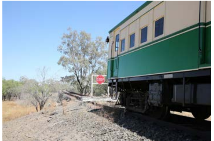
CPH 1 stands at the Walgett Silo stop block. The bridges beyond are unsound. Photo Robert Spencer
