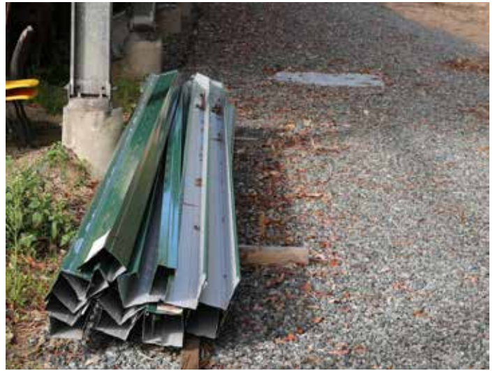
New guttering awaits installation (note the gravel formation in place for No. 4 Road)
