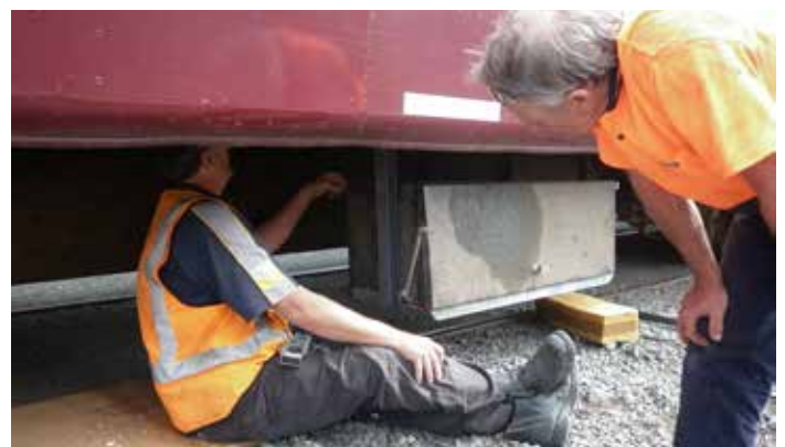
Our boilermakers fit a storage box beneath 721
