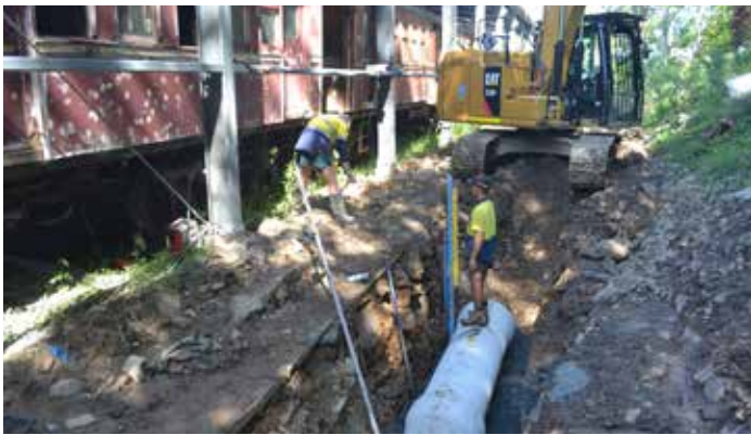
Pipe laying in progress
