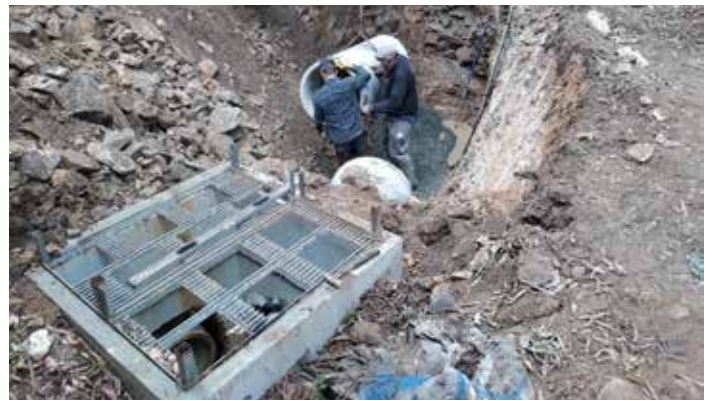
Further pipe laying. Note the presence of excavated rock.
