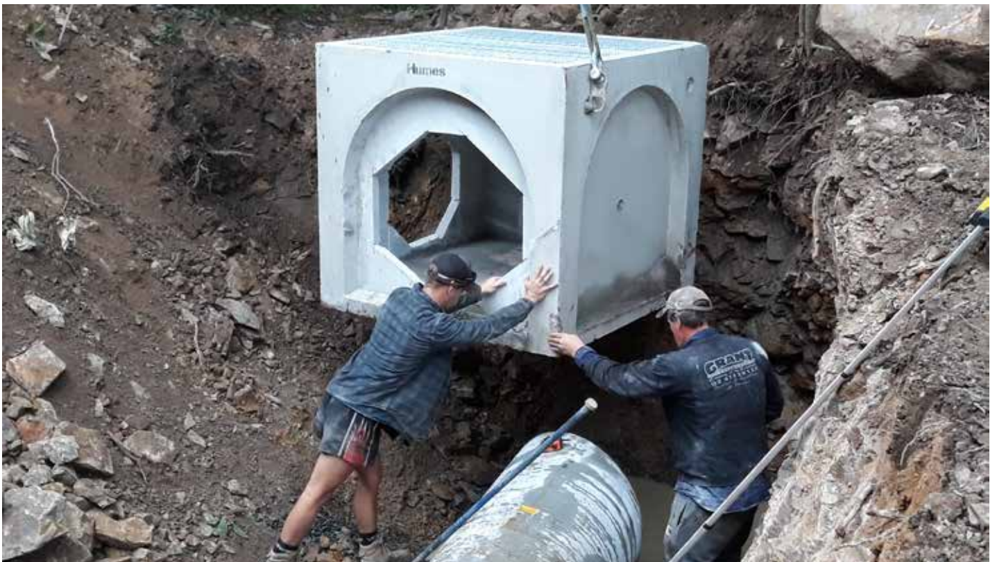
Pit being installed
