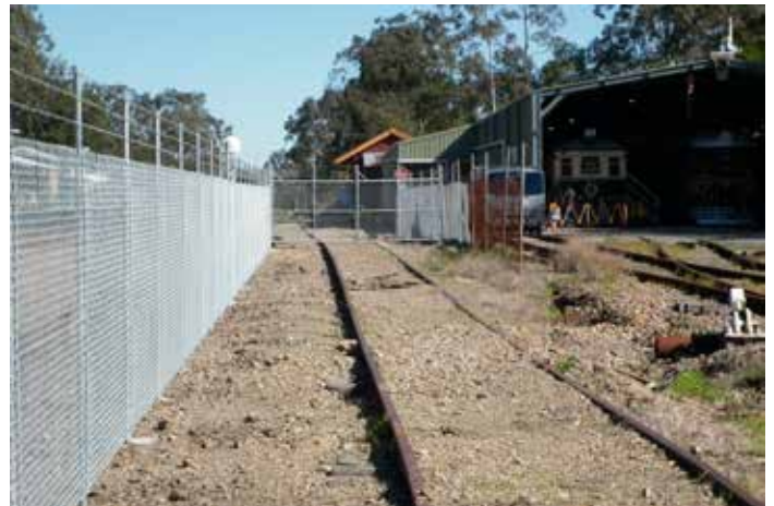
New fencing now encloses the former abandoned siding
