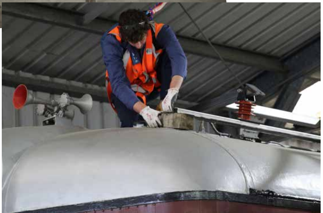
Right: Australian Rail Technology personnel install the pantograph cradle at Paterson
