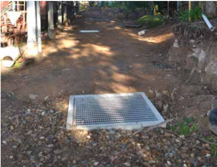
Final grading complete
