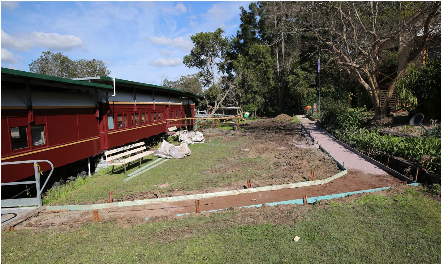
Below: Construction works for new concrete paths, 15 Aug 2022
