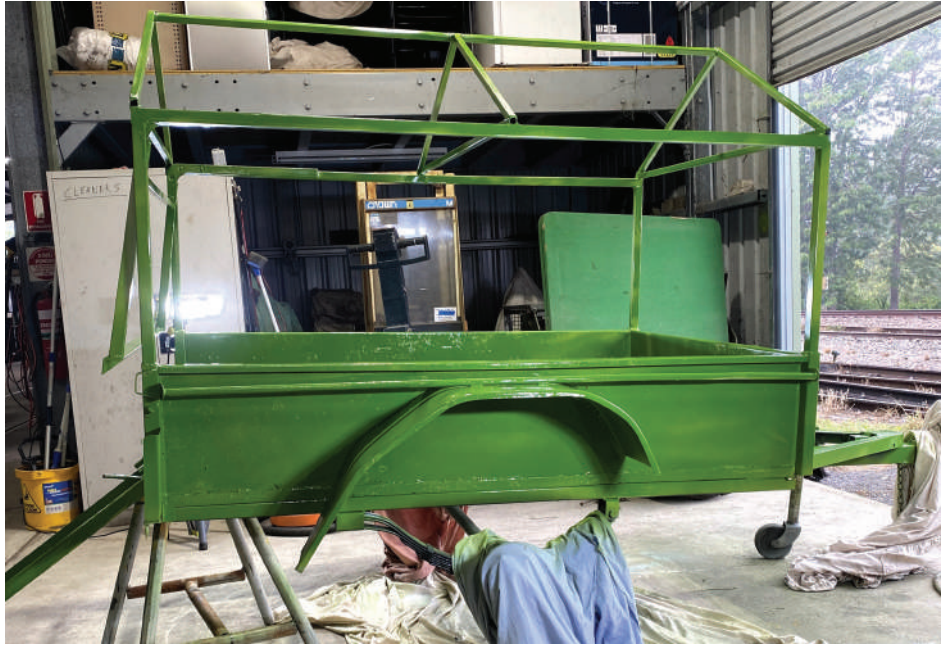
Above: Fuel trailer in an early stage of construction, 4 Jul 2023 (Allan Beard) Below: Completed fuel trailer, 22 Nov 2023 (Robert Spencer)
