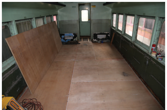
Newly laid floor sheets in 707, March 2023
