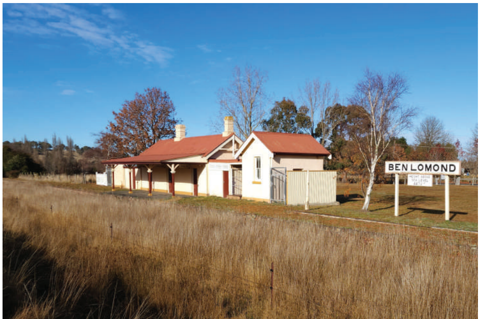
On the return to Armidale the coach followed the closed Northern Line where possible, pausing here at Ben Lomond Station, which is bathed in glorious afternoon winter sunshine, 12 Jun 2023
