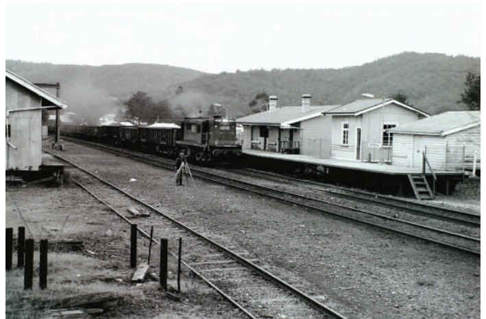
Mick Turton commences the property boundary survey utilising the permanent railway survey markers as a starting point.
