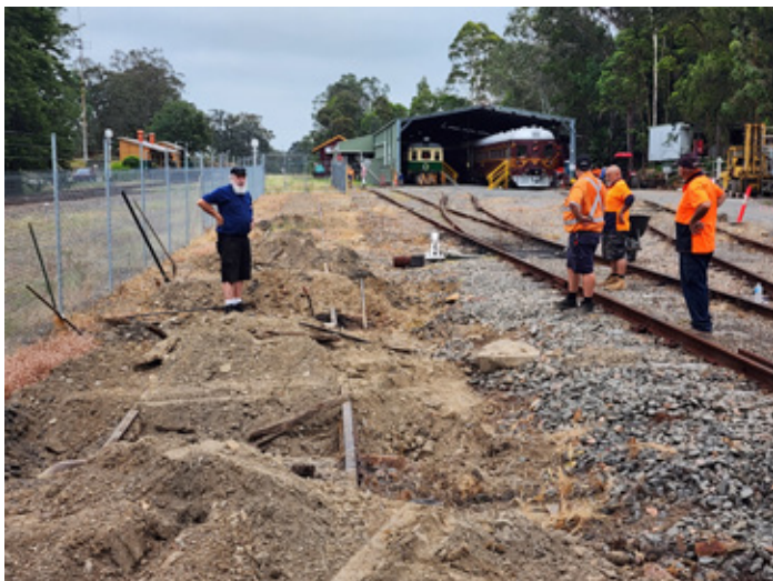
Work is underway to refurbish the former disused siding, 6 Nov 2024.
