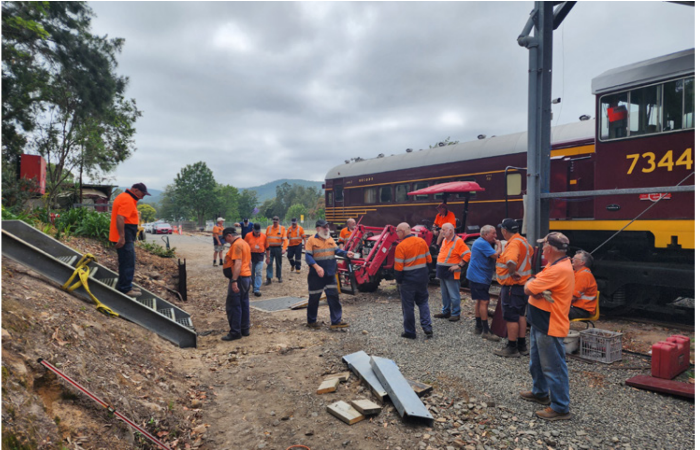
Curious onlookers watch the new steps being installed.
