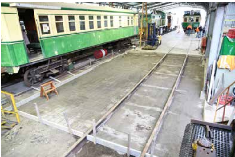
The carpenter's bench, and later the work platform it sits upon, are removed so the concrete floor can be extended further into the Main Shed. [TRMS]
