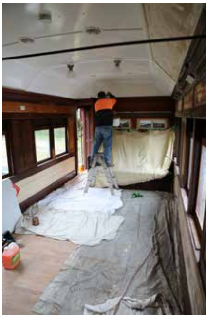
The walls and ceiling in the BR car's kitchen/lounge area have been sanded and painting is well underway. [TRMS]
