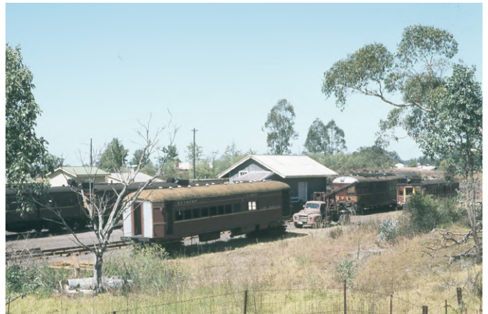
The site as viewed from Webbers Creek Road
