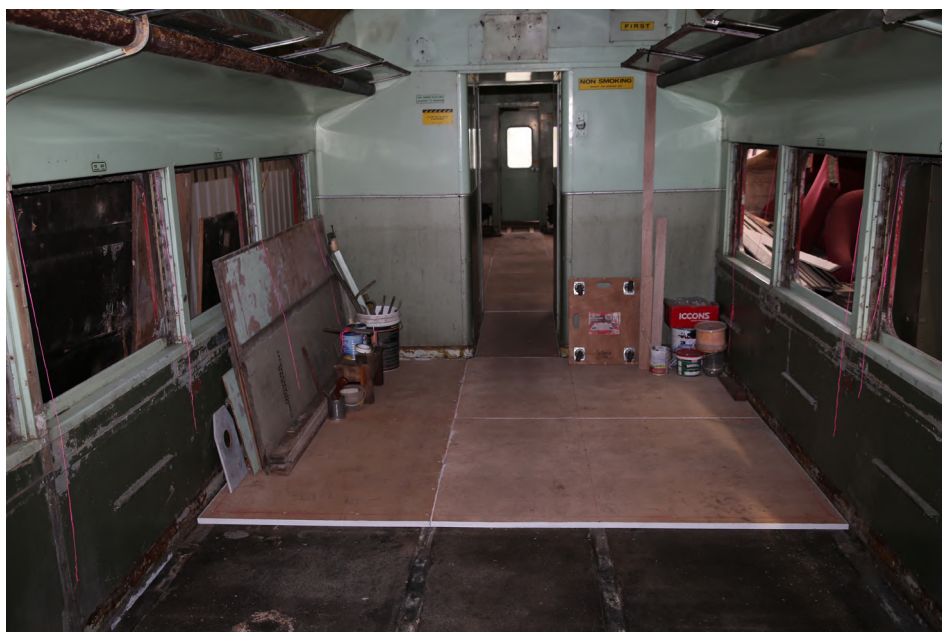
The interior of CT 702 showing newly laid floor
