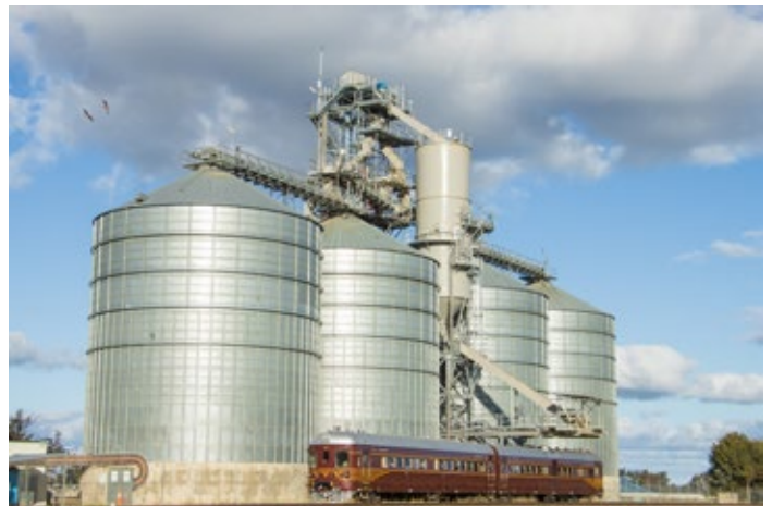
621/721 is dwarfed by grain silos in Red Bend Railway Yard (south of Forbes), 10 June 2024 (Phil Smith)
