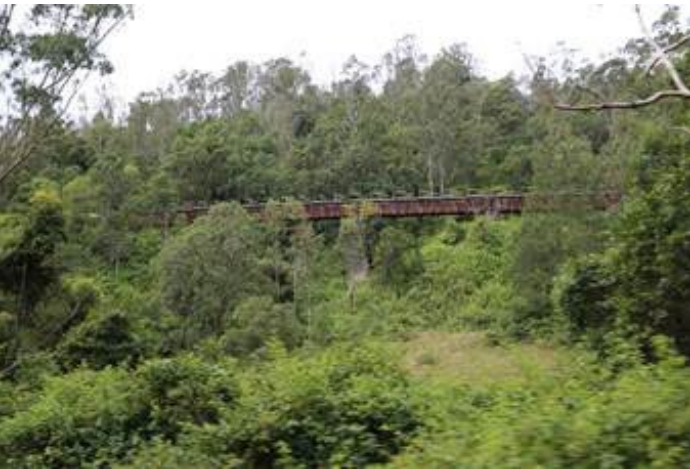
A bridge in dense forest on the upper level of the Border Loop Spiral. 621/721 has crossed this bridge, travelling from left to right. The track then spirals 360 degrees, including through two tunnels in the hill behind the bridge, to emerge on the lower level where this picture was taken, 621/721 again travelling from left to right of the picture, toward Kyogle (R. Spencer)
