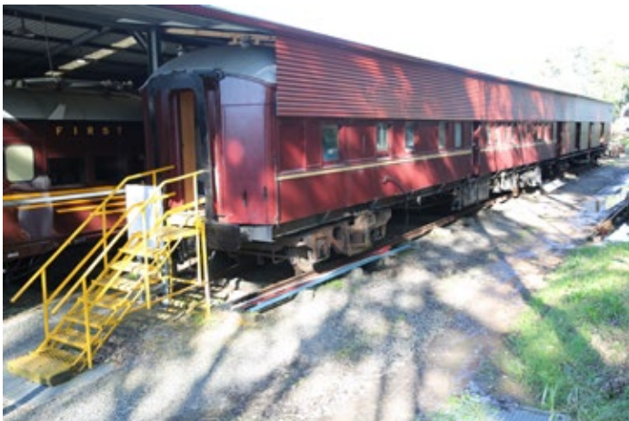
A new roof protects the FZ and MHO carriages. The FZ has improved step access.
