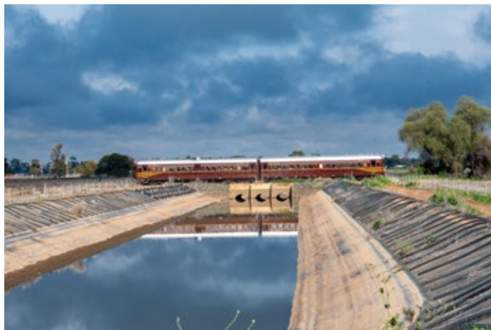
Narromine water scheme crossing 9 June 2024 (Wayne Coleman)
