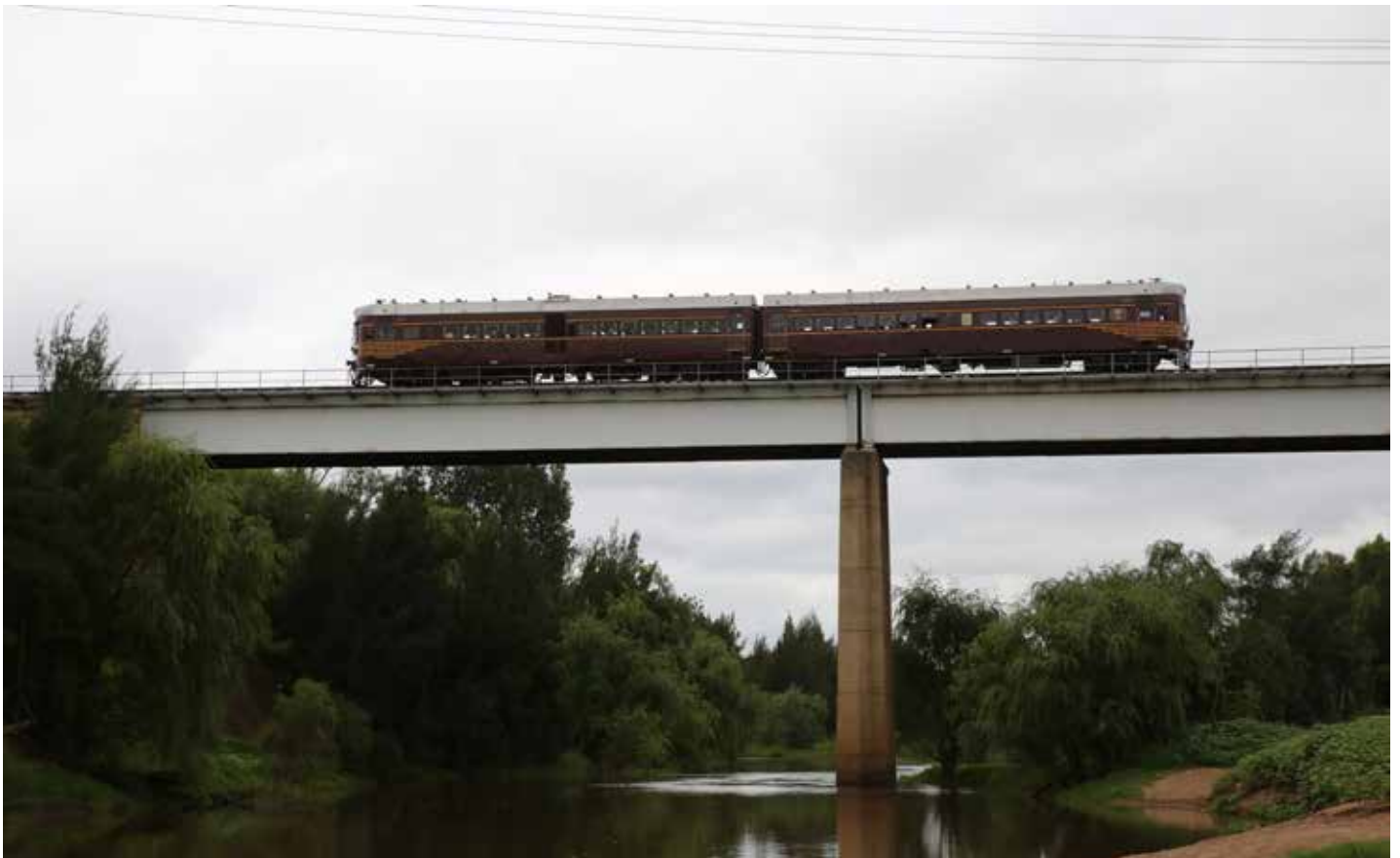
Below: 621/721 crosses the Hunter River at Singleton, 27 Feb 2021 (Robert Spencer)
