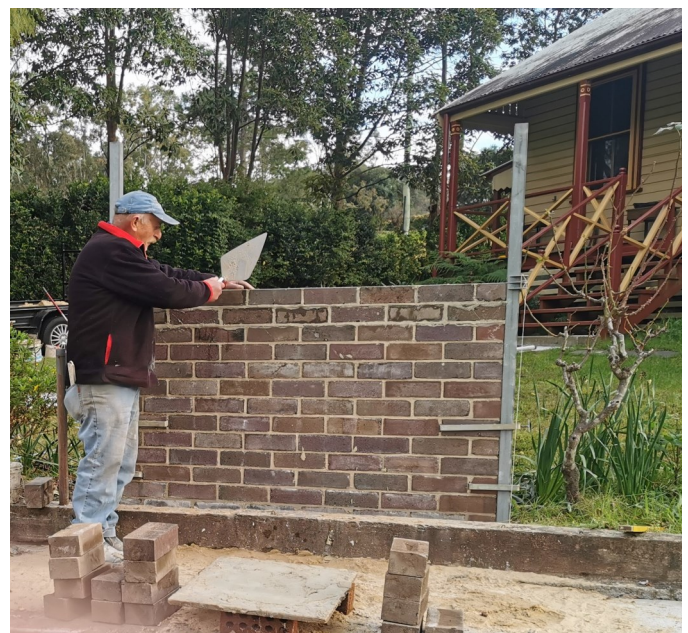
Greg Duncan is seen here constructing the memorial wall (Graeme Holloway)
