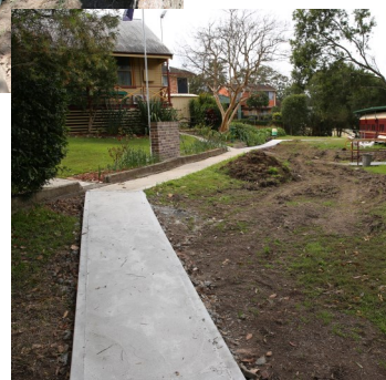
New concrete paths now extend beyond those laid earlier this year
