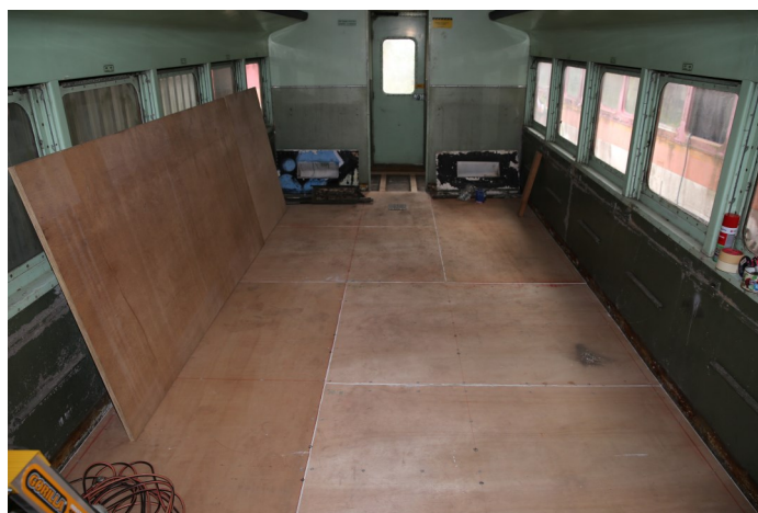
Newly laid floor in 707, 20 Mar
