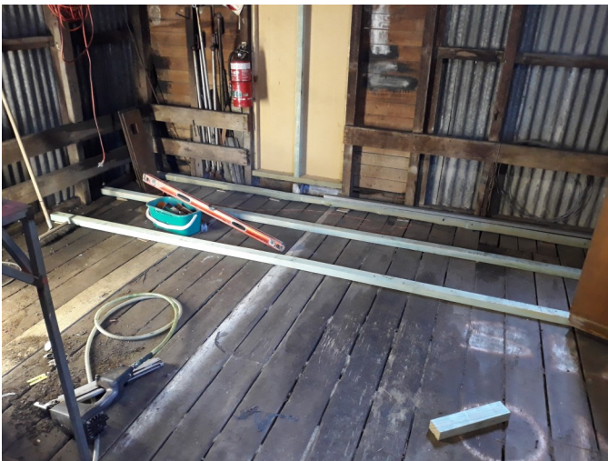
The first battens are laid – 28 August. Photo: Bruce Agland
