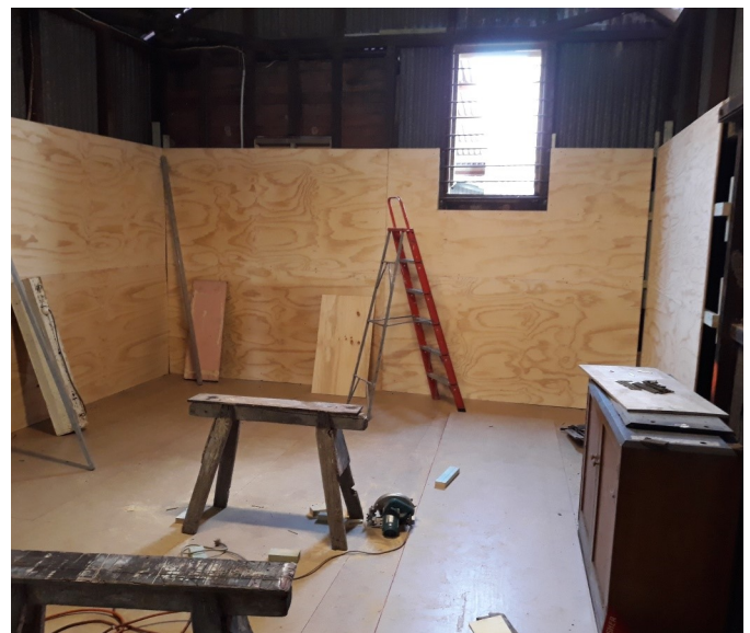
Work is well under way on 11 September. Photo: Bruce Agland
