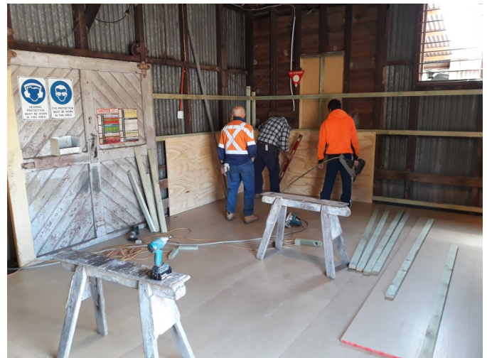
Kevin and his team installing wall sheets. Photo: Bruce Agland
