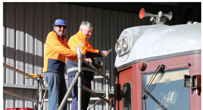
Ted Dunbar and Warren Mills waterproof 402's roof with Emer-Clad
