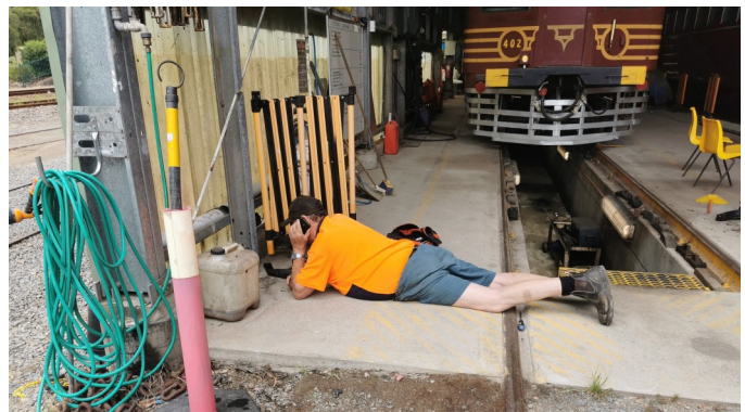
Multi-tasking, Bruce Agland secures the safety barrier in place whilst working the phone
