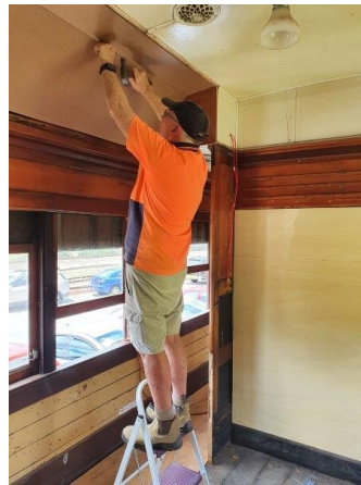
Ray Kildey at work in the new BR lounge
