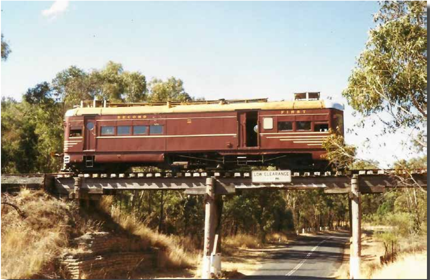
Left: HPC 402 crosses over the main road between Coonabarabran and Yearinan, Oct 1994. This bridge has since been removed.
