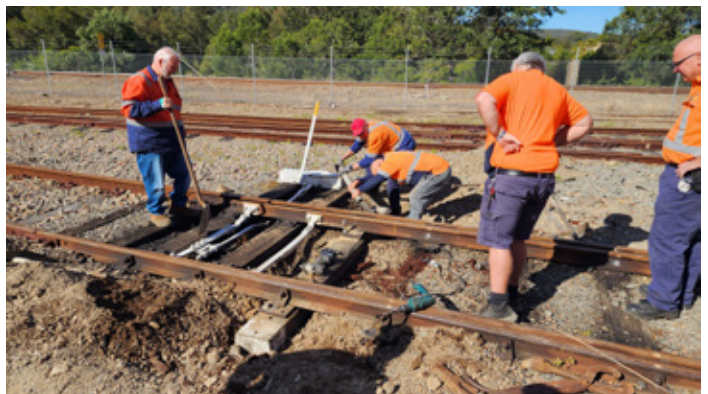
Timber sleeper replacement beneath points leading to 2 and 3 roads, June 2025
