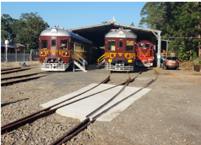
Concrete crossing for improved traffic access to the shed
