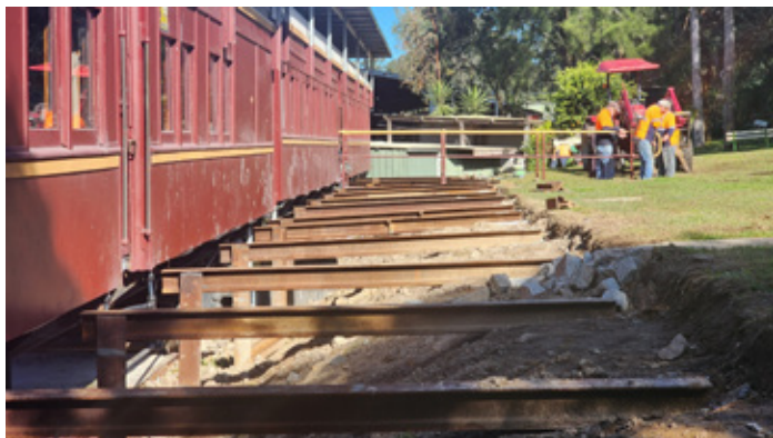
Construction work is underway to create a platform beside the TAM and BR carriages, 18 June 2025
