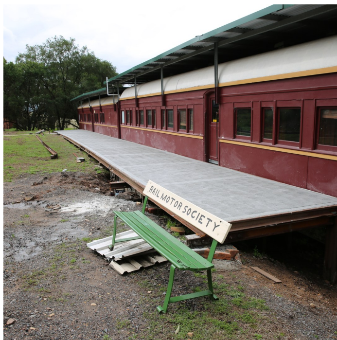
The newly poured concrete platform beside the TAM and BR carriages
