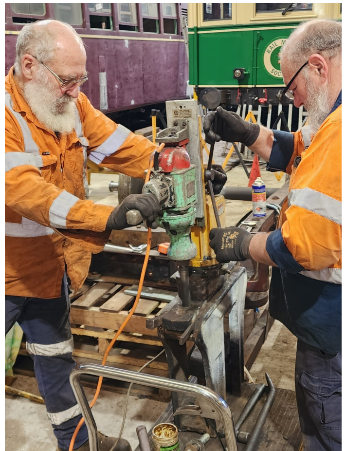
Ross Goodman and Mark Bennett operate a drill equipped with a powerful magnetic base to enlarge old rivet holes to accept new bolts in a CPH bogie frame
