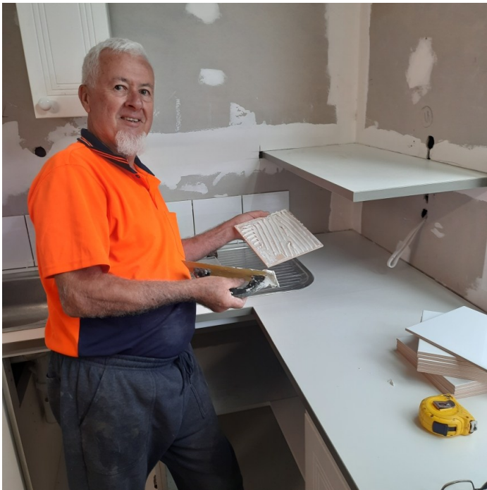
Tony Price affixes tiling to the kitchen walls in the new meal room
