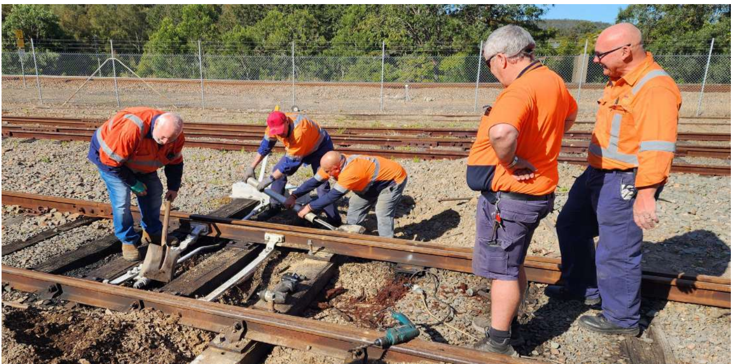
Timber sleeper replacement in the depot yard under close supervision!
